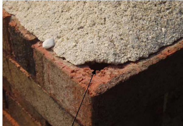
Chimney cap hole needs proper sealing.
